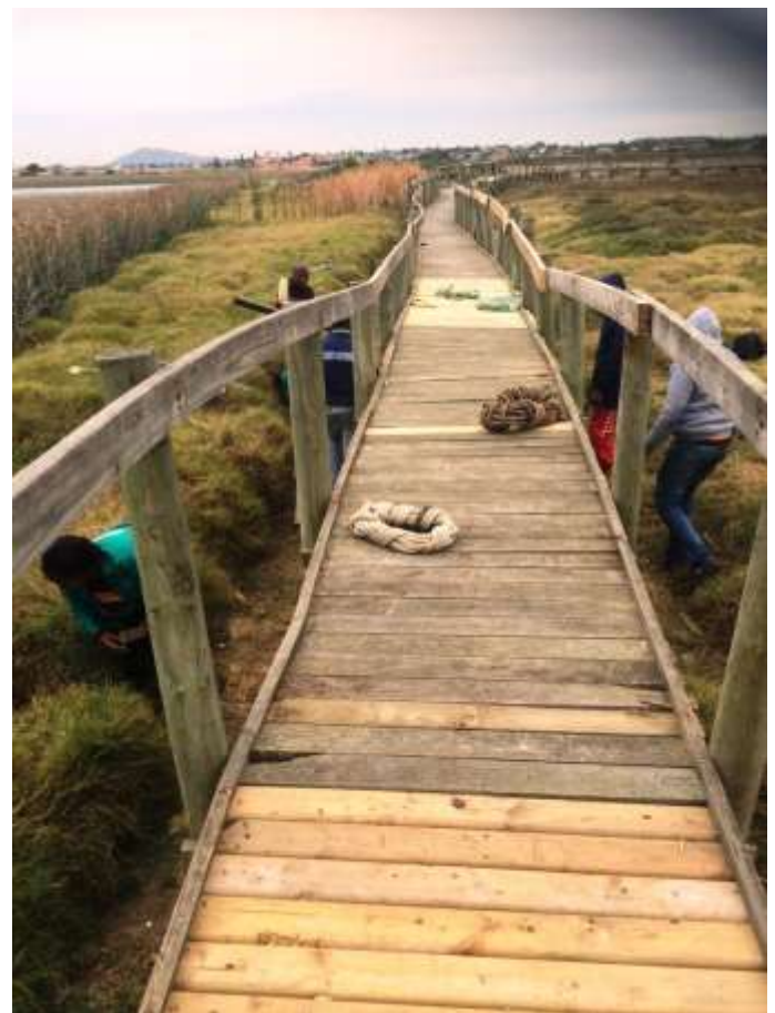
Figure 34. Boardwalk repairs under way.
